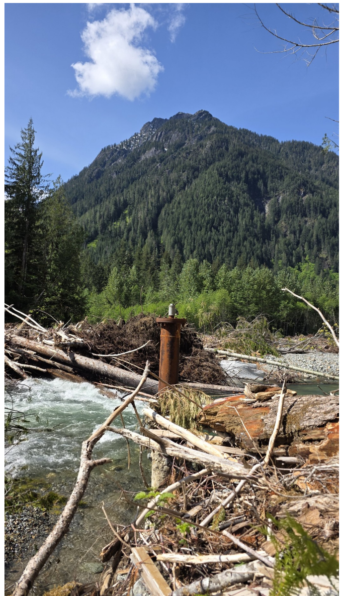
Figure 1: Geothermal exploration well drilled by Snohomish County PUD in 2011. Prior to the 2025 flood, the well was located within a forested area adjacent to historic cabins. Today, river migration has swept over the mineral springs and left the wellhead exposed within the active flood channel.
